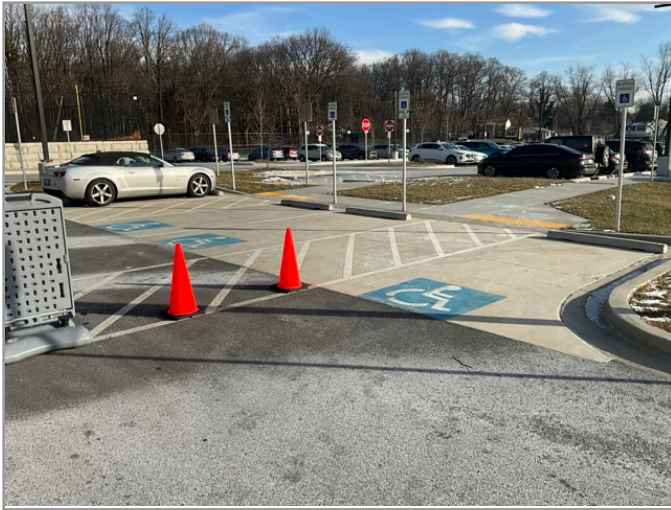
OVERVIEW OF ACCESSIBLE PARKING AREA
