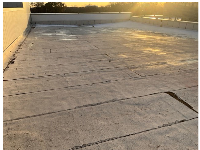
6 - PRIMARY ROOF OVERVIEW
